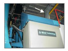
All cables running between this 8 section M-2000 Electronic Timing System in the control room and the I.S. Machine are contained in the small wireway above the machine Junction Box (Note the arrow). Only five (5) small data cables and one power cable are required. This greatly reduces cable and wireway costs as well as the installation time and space requirements for large cable trays.
